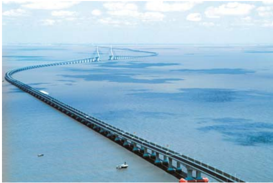
Donghai Bridge to Deepwater Harbor Yangshan Island
